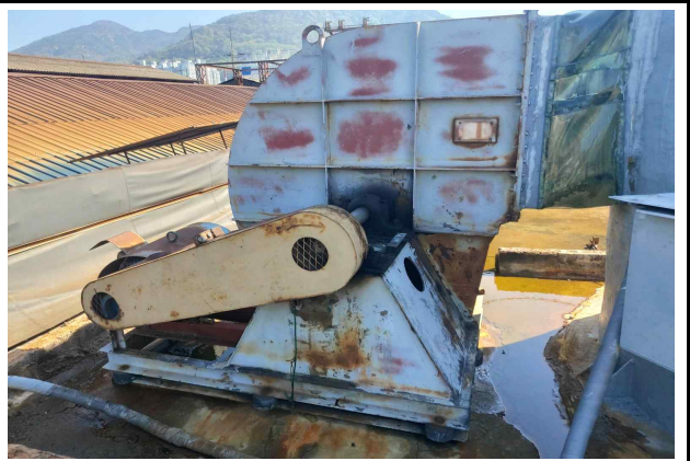
Fan Shaft Bearing Oil 누유
